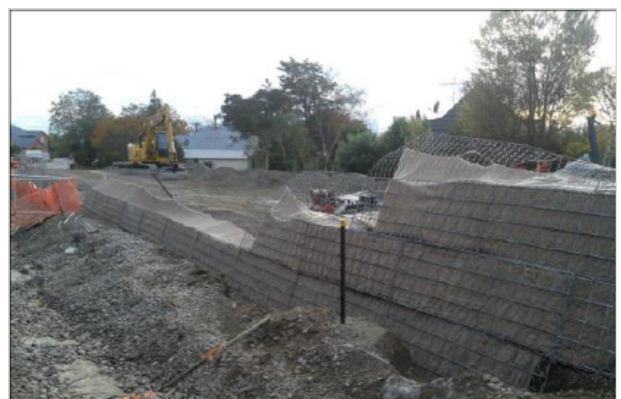
GTM embankment: Installation of GTM cage in progress
