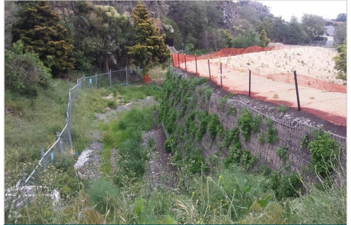
GTM embankment: Construction completed & vegetation growing on GTM face
