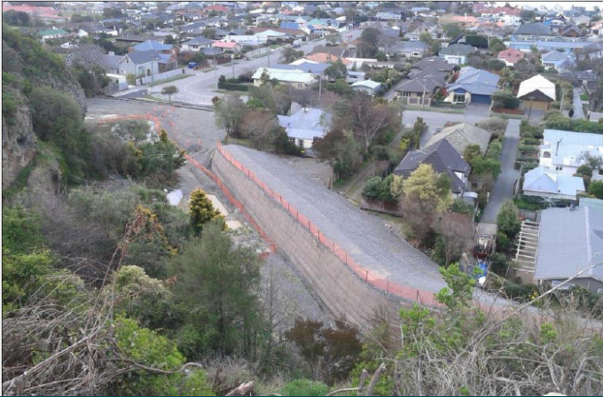
GTM embankment: Construction completed
