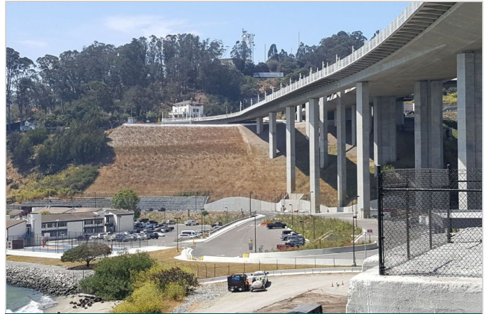
Achieved vegetated slope
