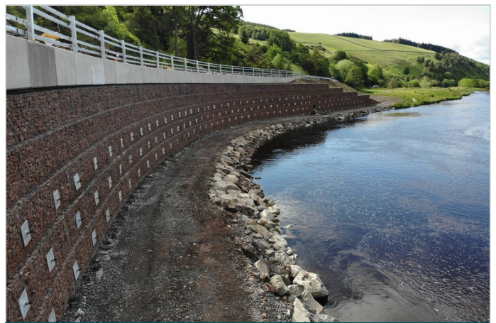
Completed retaining wall
