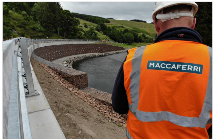
Our UK Construction Manager and the completed works
