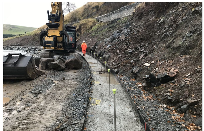
Foundation preparation for the hybrid reinforced soil wall
