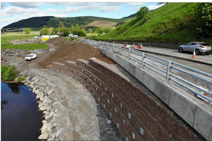
Gabion Terramesh in position
