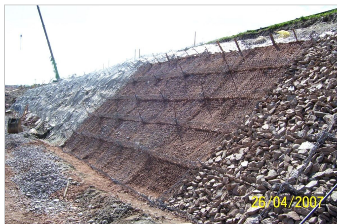
Geomac during installation showing partially filled units
