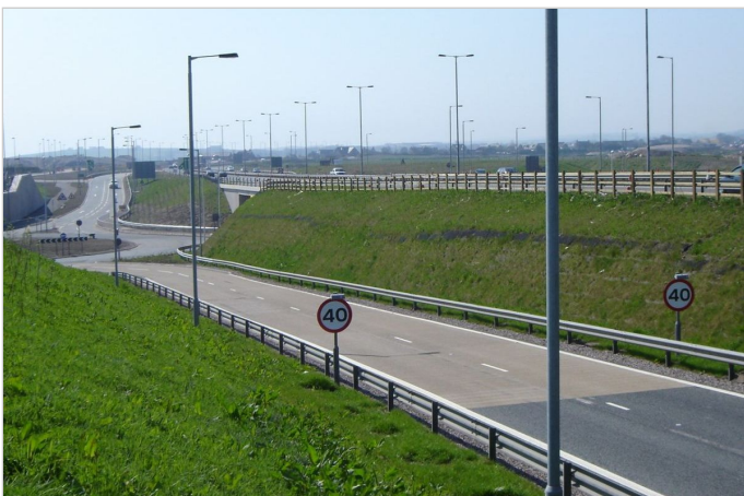
After construction, showing successful vegetation
