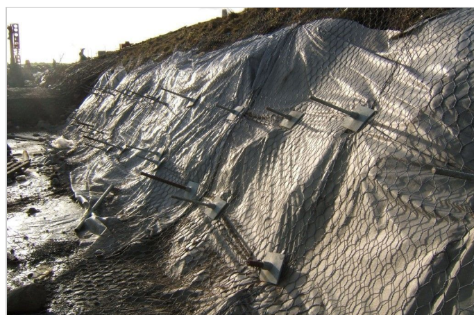
Empty Geomacs, placed on soil-nailed slope
