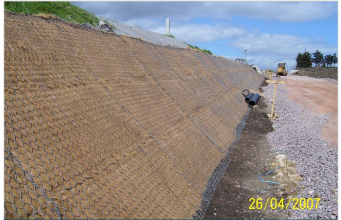
After installation, prior to vegetation establishment
