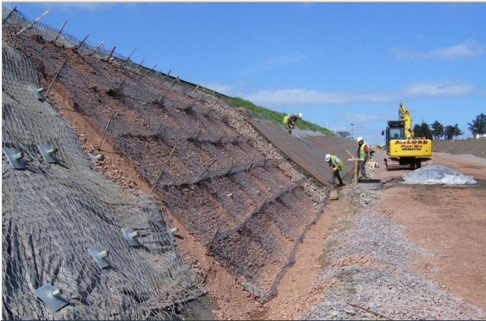
Geomac during installation
