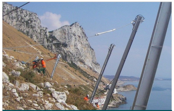
Erecting catch fence posts / drilling anchors
