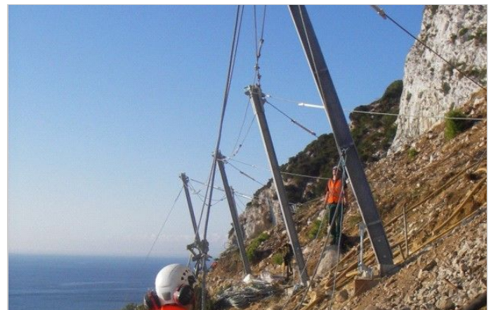
Raising catch fence posts into position
