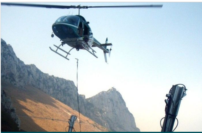
Using helicopters to lift posts into position
