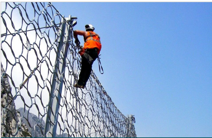
Securing main absorption panels to upper cables and posts
