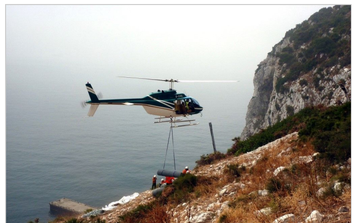
Rolls of debris mesh being lifted to project site
