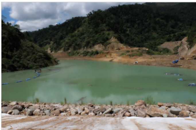
September 2016 - During Construction
