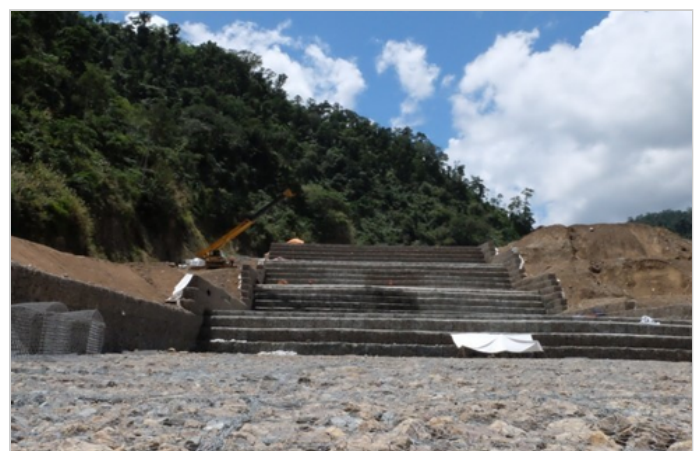
September 2016 - During Construction
