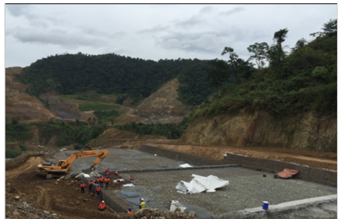
July 2016- During Construction
