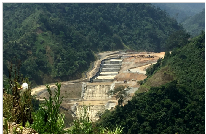
September 2016 - During Construction
