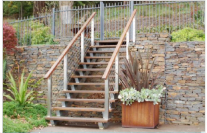
Stairway Within Gabion Walls
