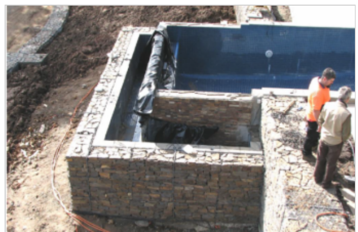
500 mm Thick Gabion Facade Around The Swimming Pool
