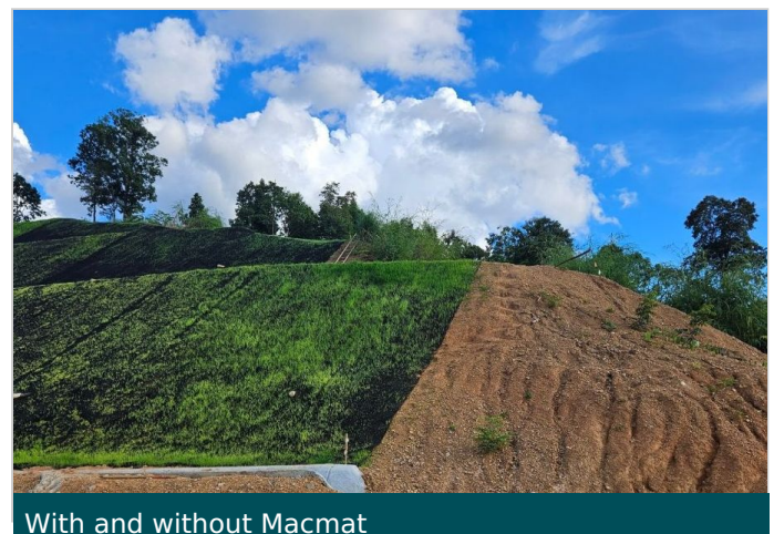
Slope Protection with Macmat
