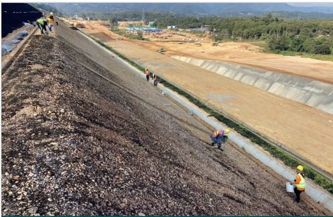
Preparation Before Installation of Macmat
