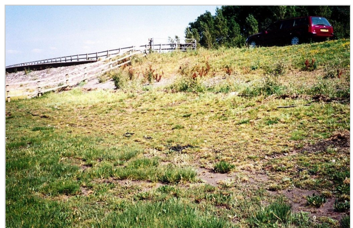
Newly installed Reno mattress / Geomac
