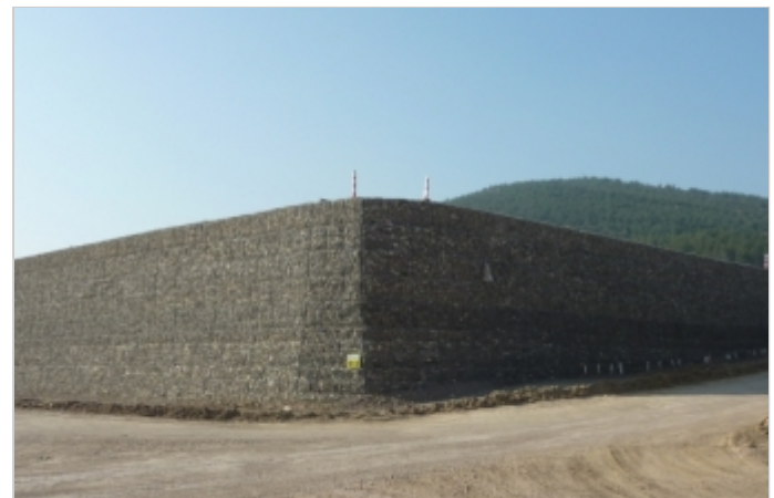
Panaromic view of Terramesh System
