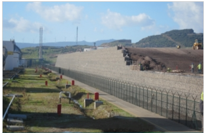
During the installation phase
