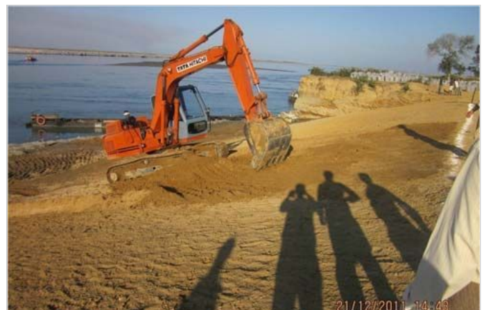
Photo 2: Dressing of slope during construction
