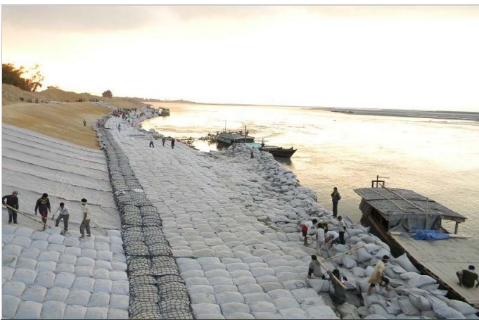
Photo 3: Placement of MacBag® on the river bank
