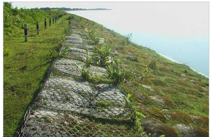
Photo 6: Condition of MacBag® after 2 years
