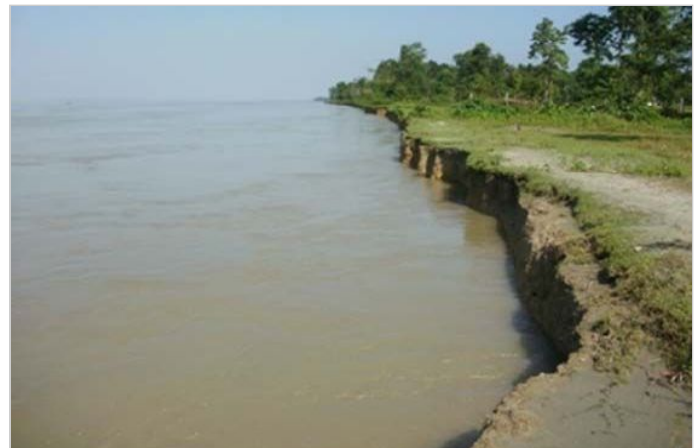
Photo 1: Scouring of the banks of Brahmaputra river
