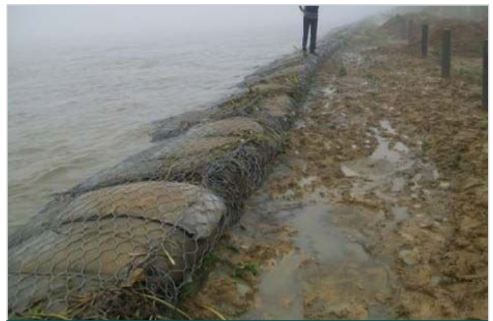
Photo 4: Condition of MacBag® and river bank during flood
