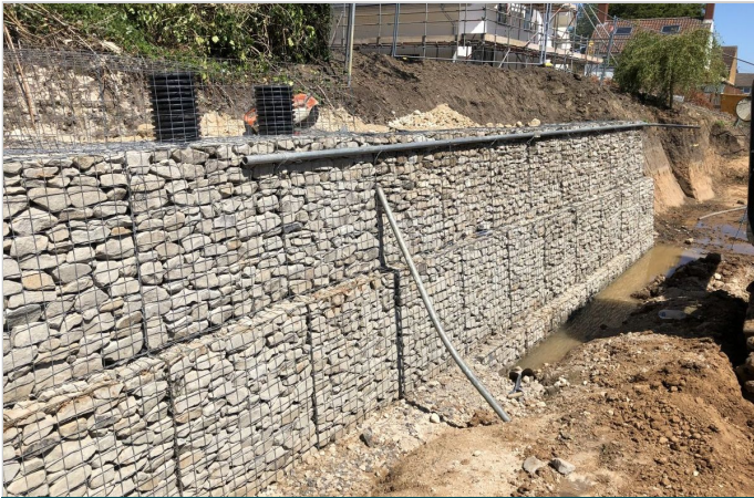
Gabions with hand stacked "dry stone wall" finish
