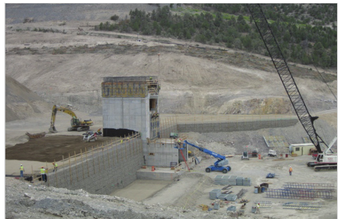
Terrawall® construction in July 2009
