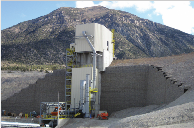
The completed Terrawall® system.
