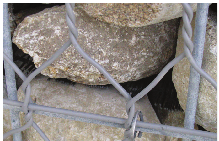
MacGrid® reinforcement is shown between the rocks which were used as filler in t
