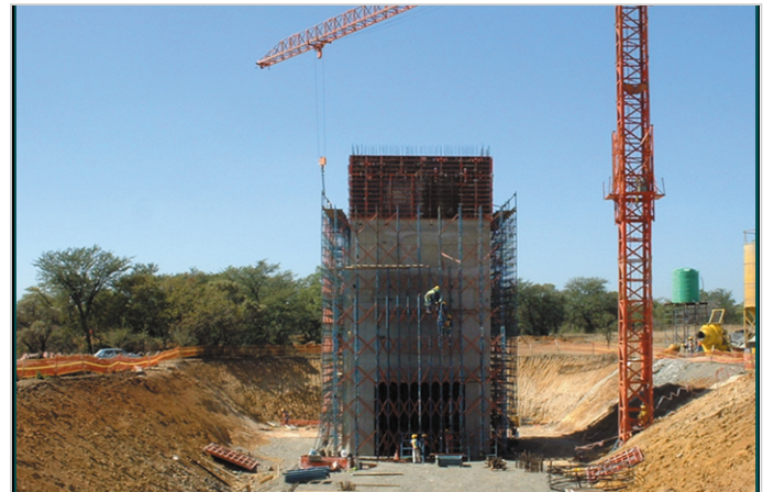
Before wall construction
