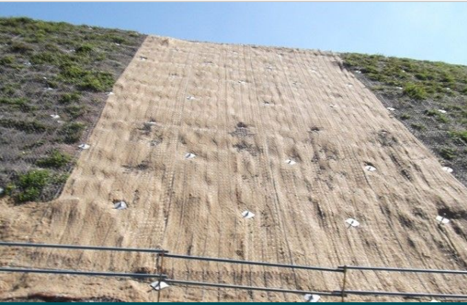
Steelgrid HR30 mesh underlain by Coir blanket
