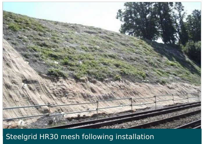
Steelgrid HR30 mesh following installation
