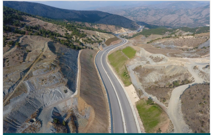
Figure 4: Highway slopes covered with Macmat R1
