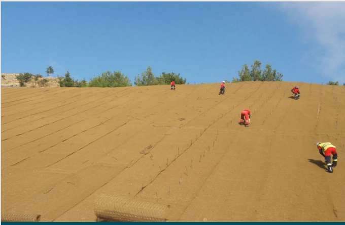
Figure 3: Quick installation of Surface Anchorages
