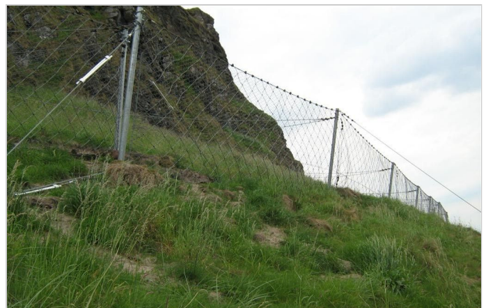
View of the catch fence installed
