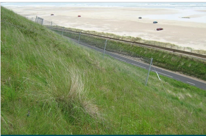
Works completed in 2011
