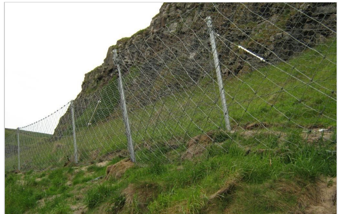
View of the catch fence installed
