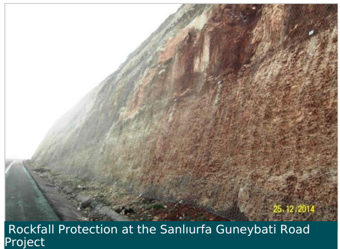
Rockfall Protection at the Sanliurfa Guneybati Road Project
