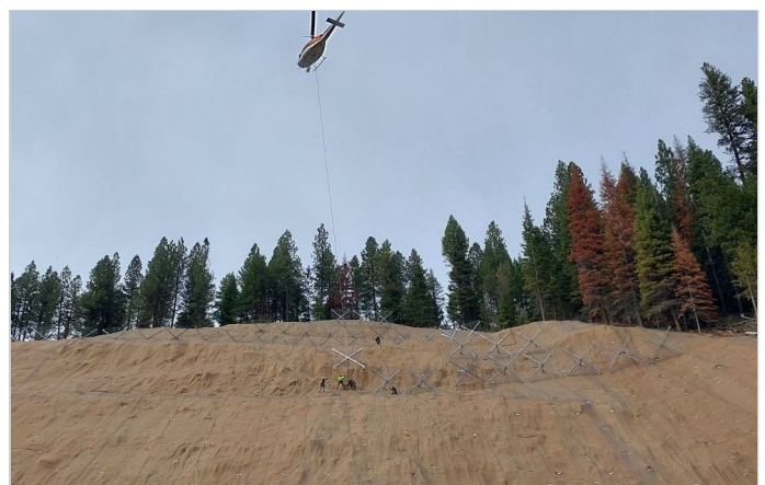
Installing Erdox Units on the slope
