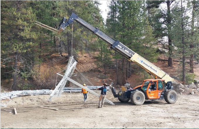
Assembling Erdox Units at the laydown yard
