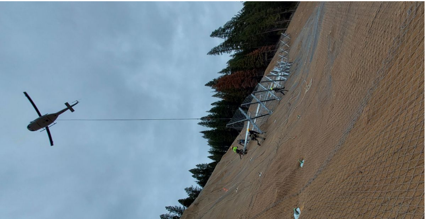
Helicopter lifting Erdox into place
