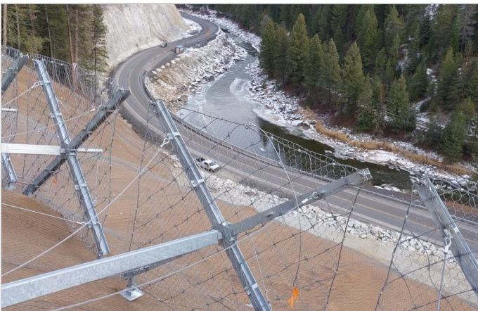
Erdox Units installed on the slope
