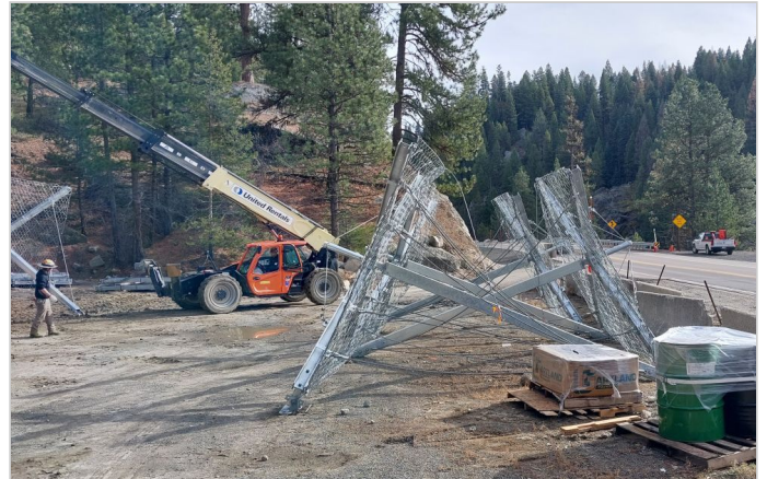
Assembled Erdox Units waiting to be flown onto the road cut
