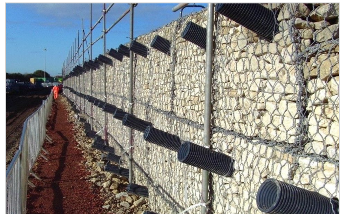
Immediately after construction, before soil nailing
