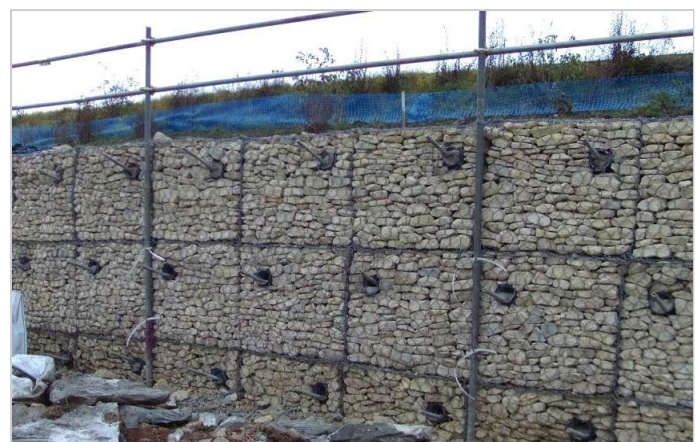
Immediately after soil nail installation
