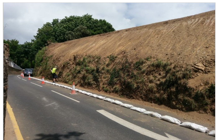
Pre-construction before the installation of MacMat® R
