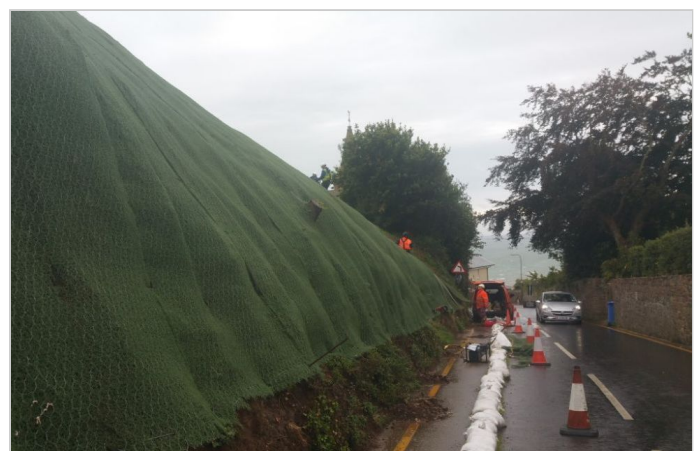
During construction in August 2016
