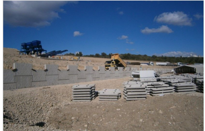
MacRes Retaining Wall Construction Phase
