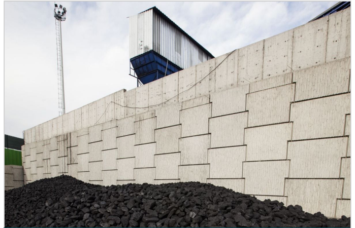
Coal Storage Area
