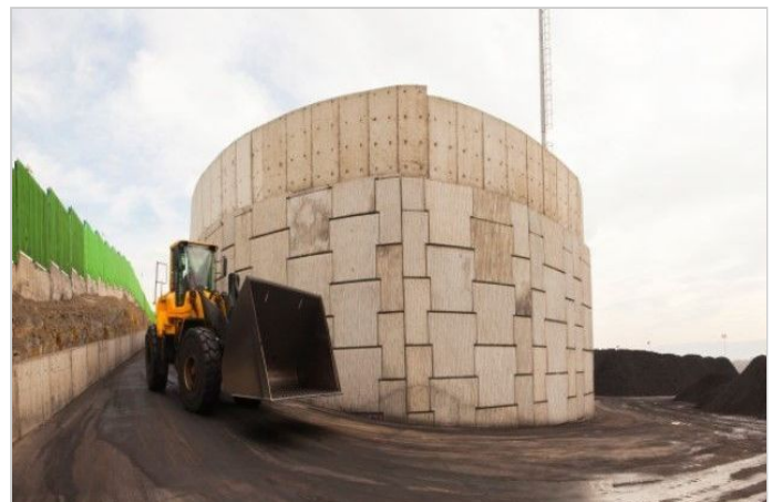
MacRes Retaining Wall
