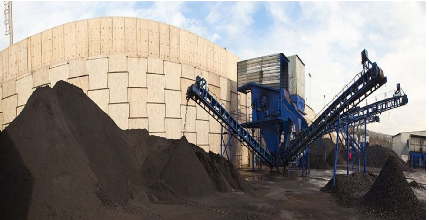
MacRes Retaining Wall
