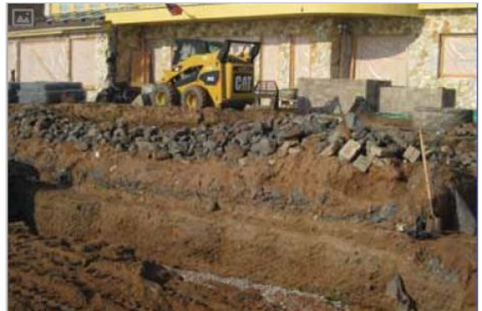
Gabion wall under construction
