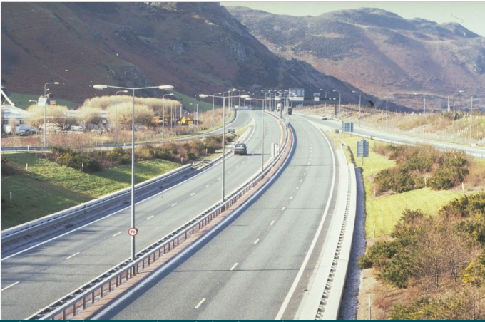
View of the completed dual carriageway
