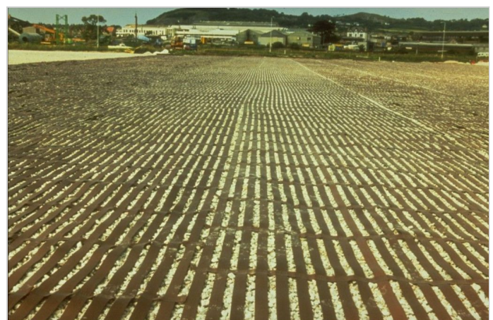
Paralink® covering the installation area
