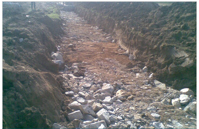
Photo 4: Foundation placing for gabion wall
