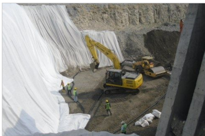
Installation of the filtering geotextile for the drainage system
