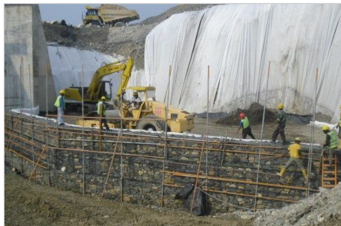
Terramesh System installation
