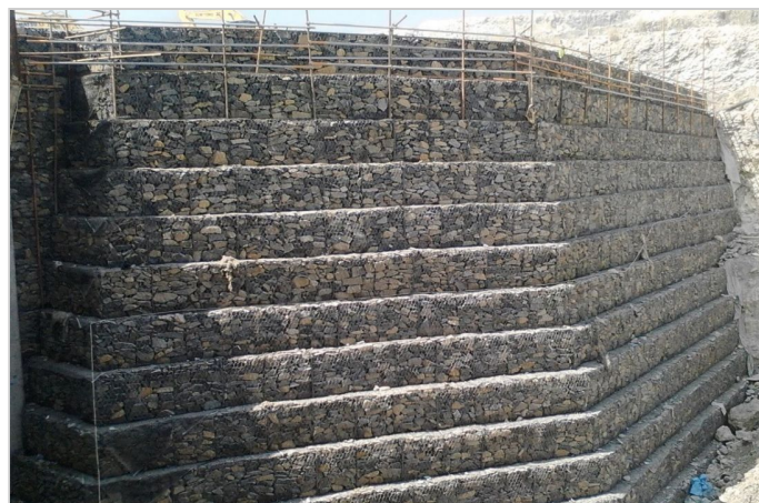
Wall after Completion
