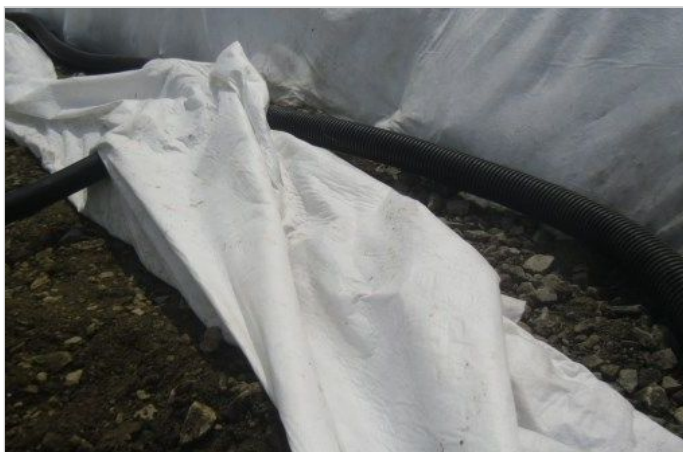
Stones as draining material; Corrugated collecting pipes
