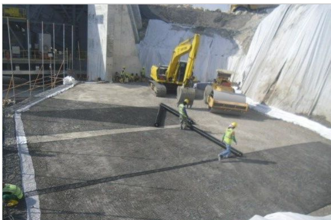
Laying MacGrid WG 15
