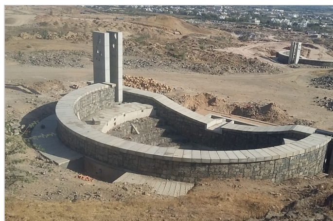
Photo 1: Series of check dams under construction
