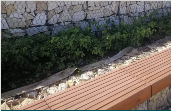
Close view of the Terramesh MSE wall with bench
