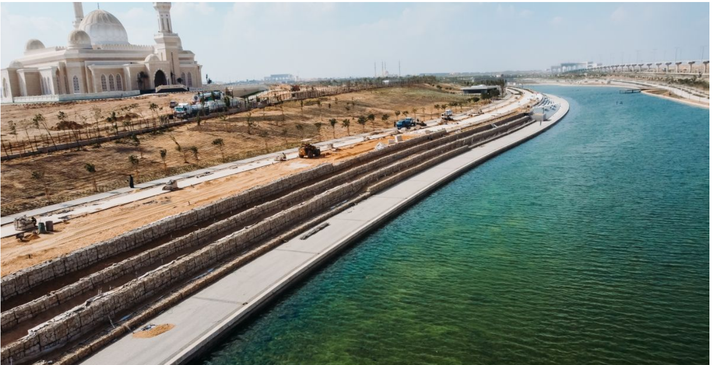
Distant view of Terramesh MSE wall along the banks of Green river
