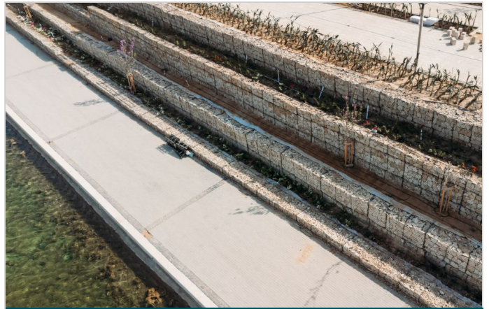
Close view of wall along Green river banks
