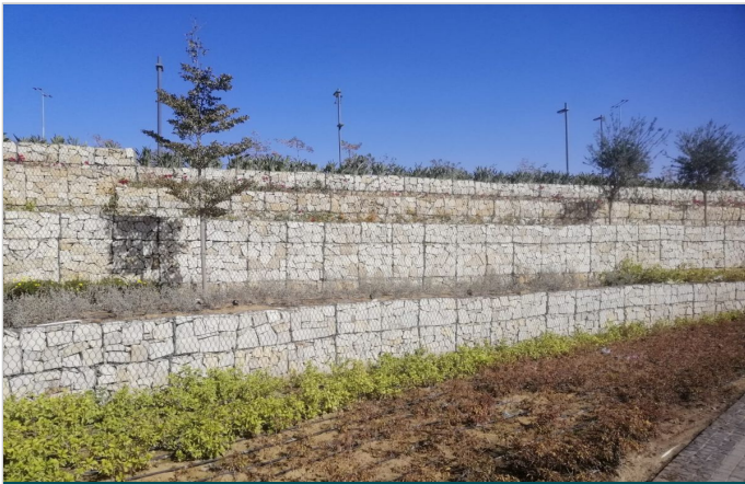
Close view of the Terramesh MSE wall with plantation
