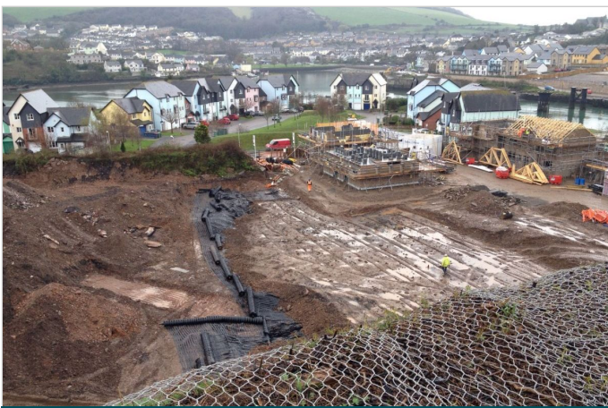
Housing construction phase starting over the ParaLink® load transfer platform
