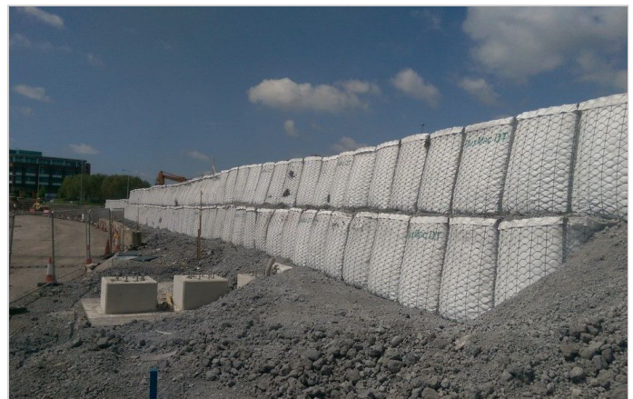
FlexMac DT temporary structure
