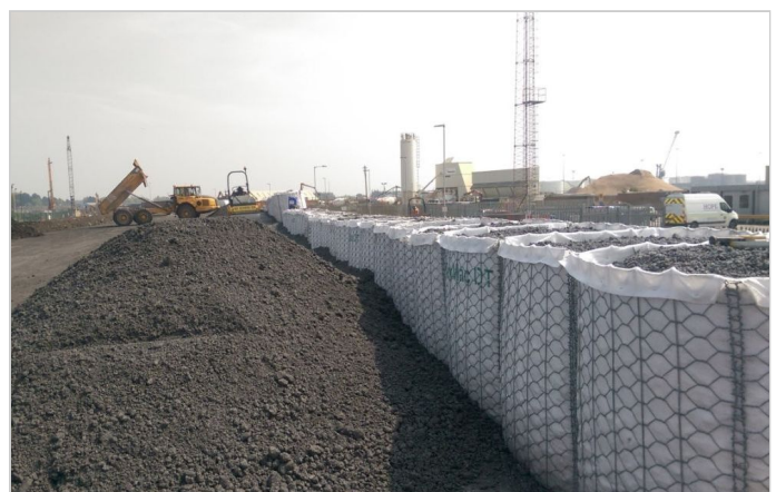
Backfill placement behind the structure
