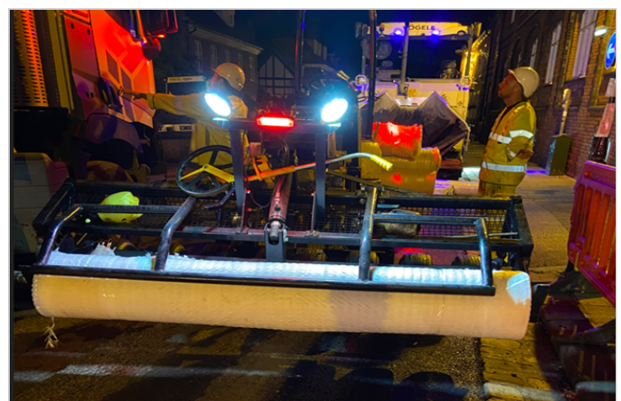
Mactex C7 is installed by specially designed Triplex Progrid plant machine
