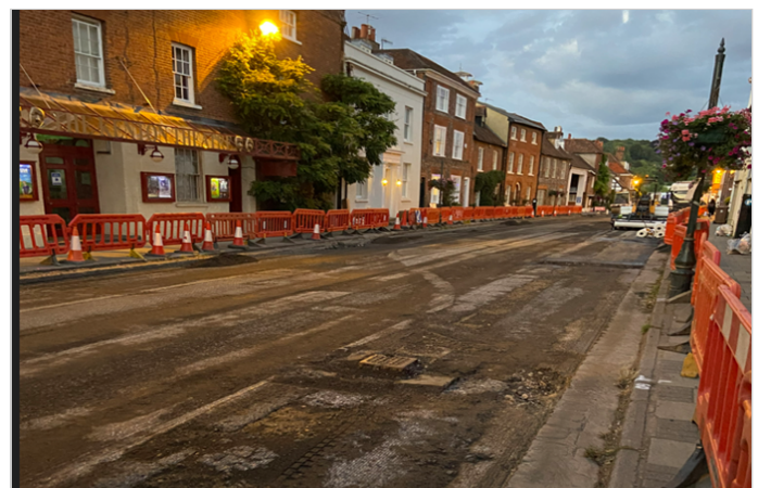
Existing surface planed off & awaiting install of Mactex C7.
