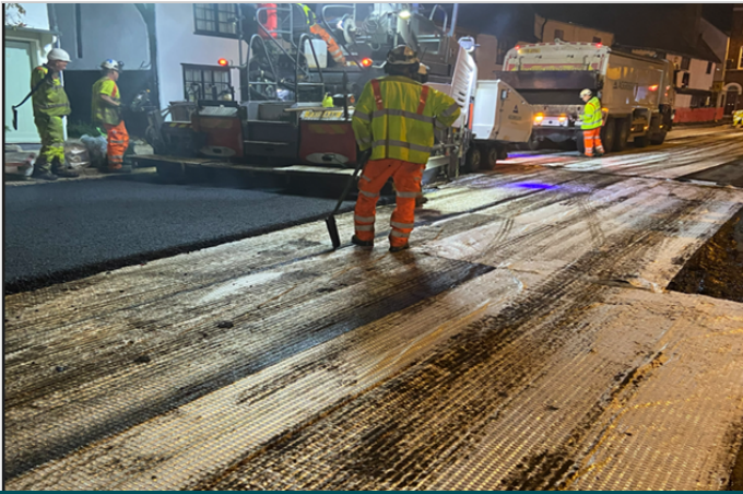
Surfacing works over the top of installed Mactex C7 10s.
