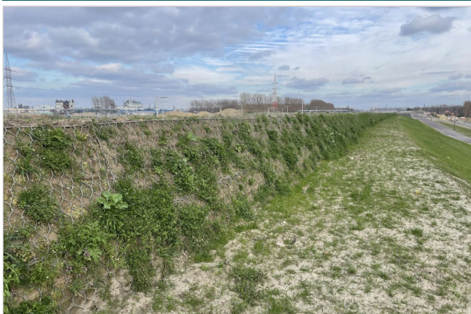
Detail of the Green Terramesh DUO elements on the top of the slope
