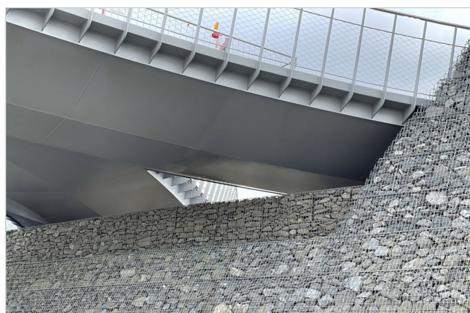
Detail of the bridge abutment
