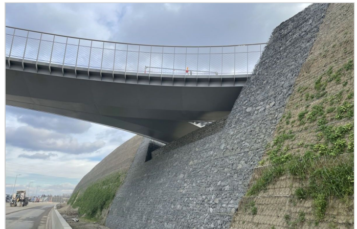
Transition between Green Terramesh and Mineral Terramesh
