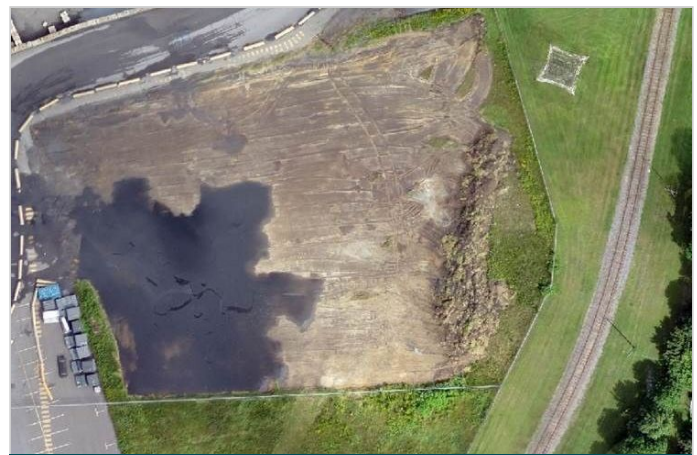
Aerial view of the land before construction
