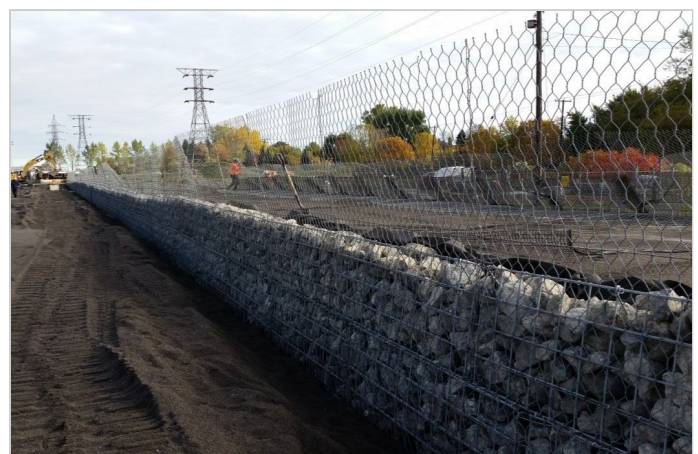
Recycled crushed concrete used for face-filling
