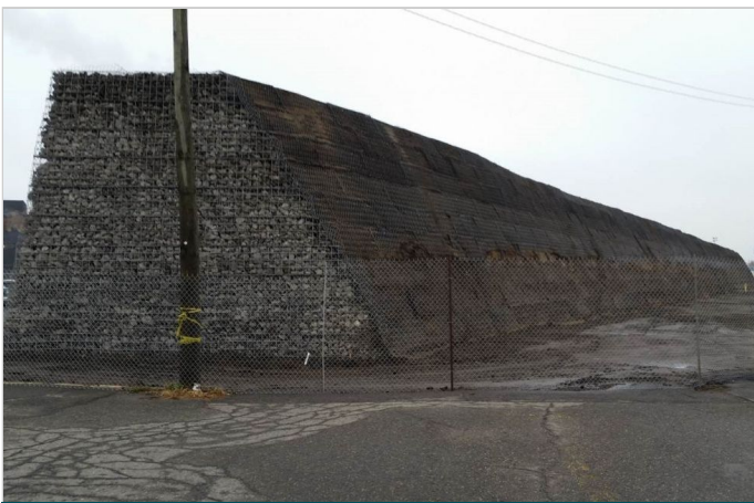
Completed city-facing side using Green Terramesh
