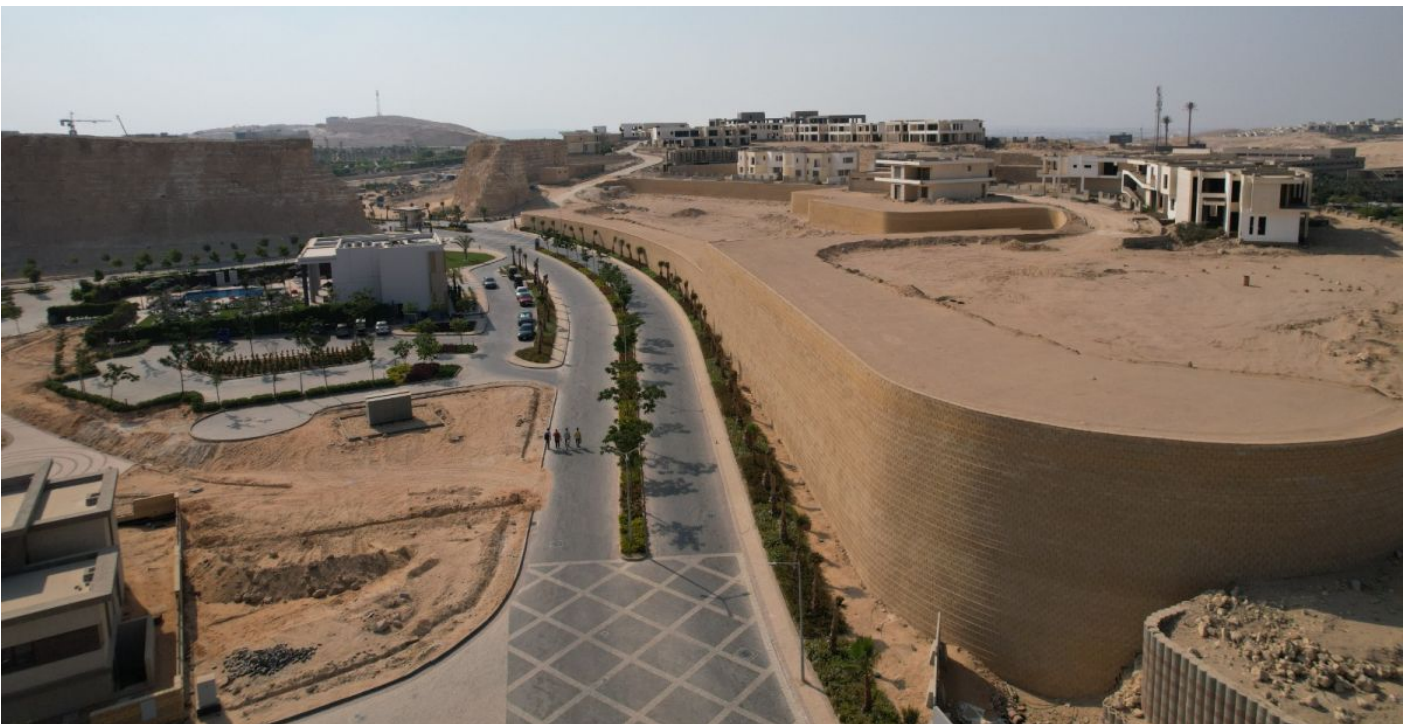
Completed high MacWall MSE wall at a critically curved location
