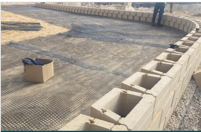
Typical details: block & geogrid
