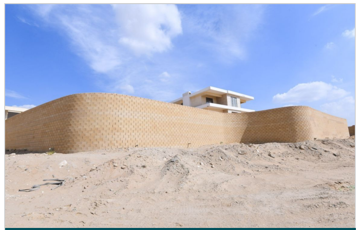
MacWall MSE wall in progress
