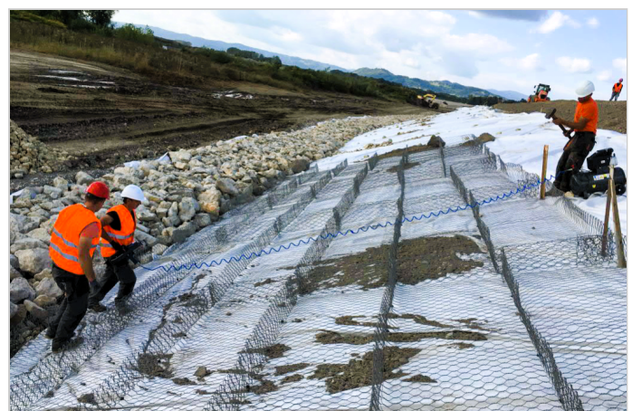
During the installation
