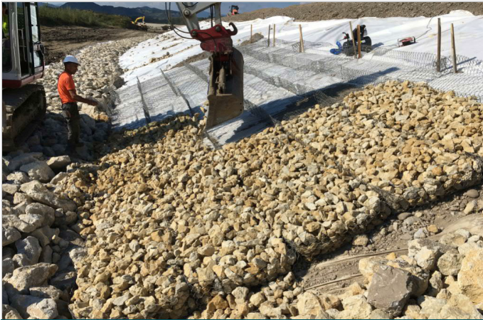
During the installation
