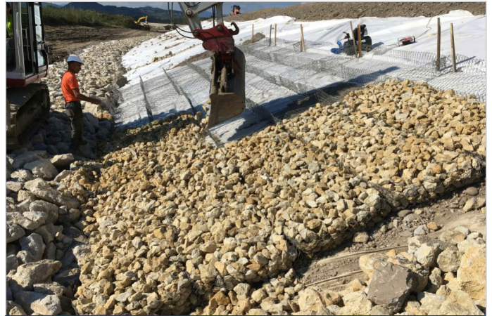
During the installation
