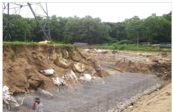
During construction (July 2007)
