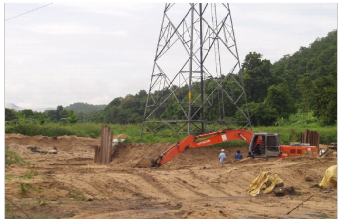
During construction (June 2007)
