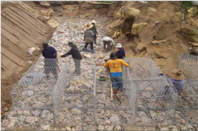
During construction (July 2007)
