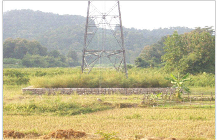
After construction (December 2007)
