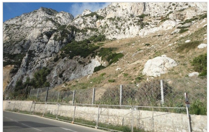
View of completed roadside barriers
