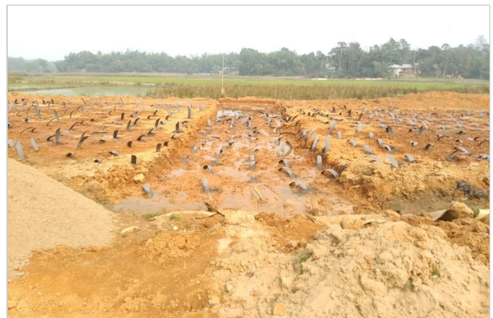
MacDrain V (PVD) installation
