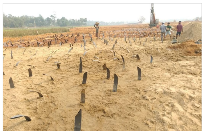
MacDrain V installation
