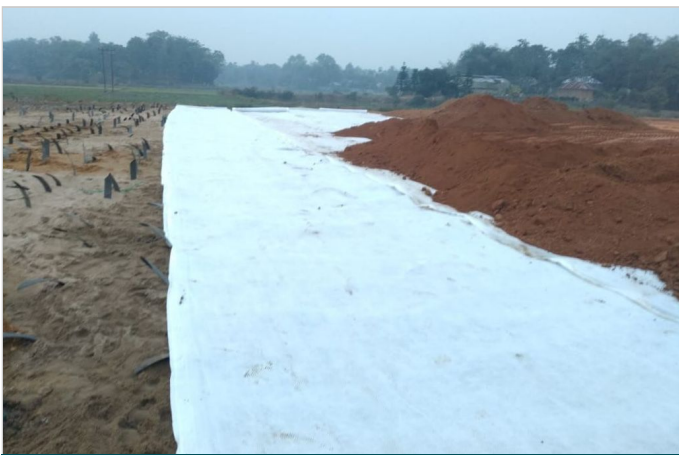
Laying of MacDrain V as drainage layer
