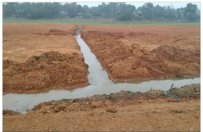
Surface drain arrangement
