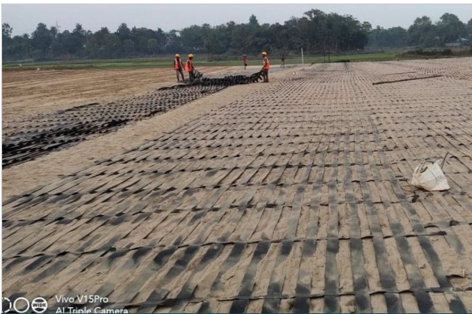
Laying of Paralink as basal reinforcement
