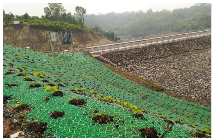
Macmat HS + Vegetation Installed
