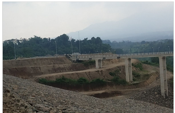
Slope Condition before Macmat Installation
