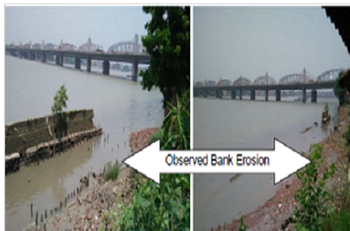
Photo 1: Severe erosion observed on the banks of river Ganga
