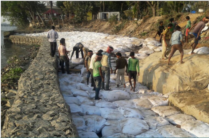
Photo 3: Placement of geotextile bags behind gabions
