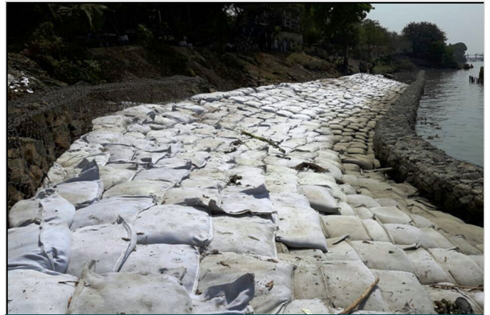
Photo 4: Installation of geotextile bags
