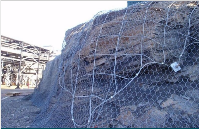
HEA panel (over RFN) securing large block on buttress
