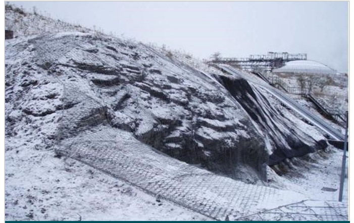
Completed installation of MacMat® R & rockfall netting
