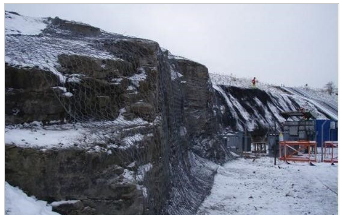
Installation in progress of MacMat® R & rockfall netting
