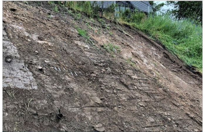
Slope face stripped of excess topsoil ahead of remedial works
