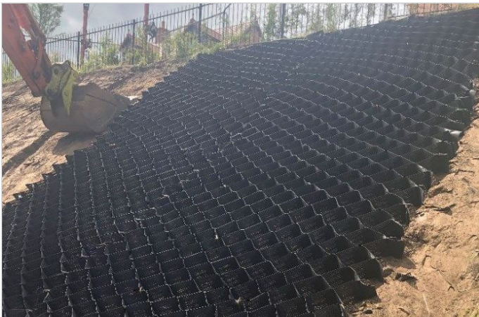
MacWeb cellular containment system ahead of topsoil filling
