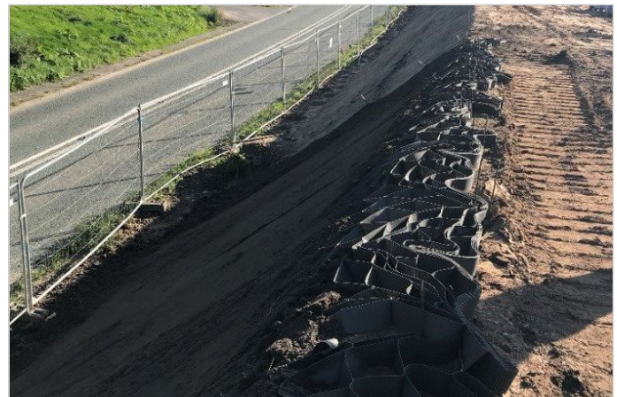
ParaGrid reinforced slope with MacWeb erosion control in 2018
