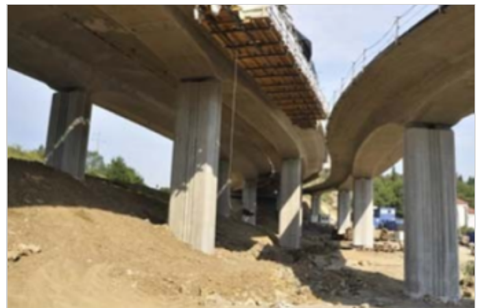
Start of construction activities
