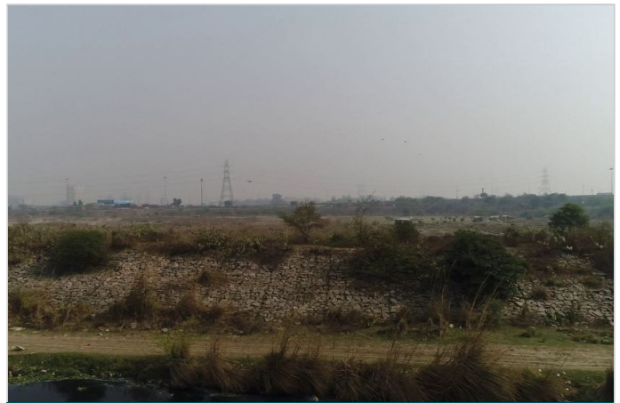
Photo 4: Completed Structure after 19 years
