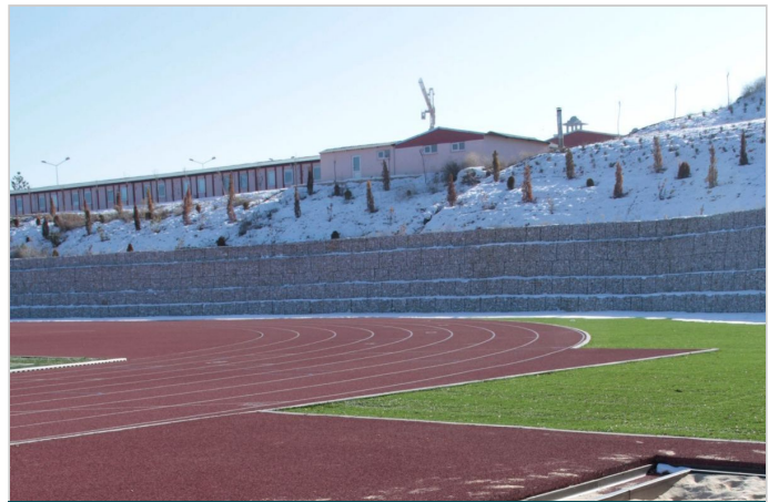
Box Gabion Retaining Wall
