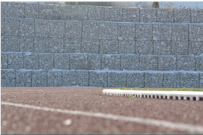
Box Gabion Retaining Wall
