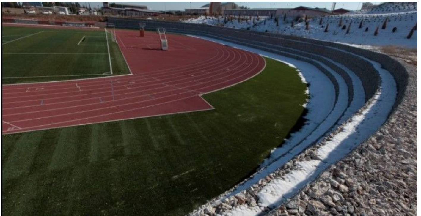
Box Gabion Retaining Wall
