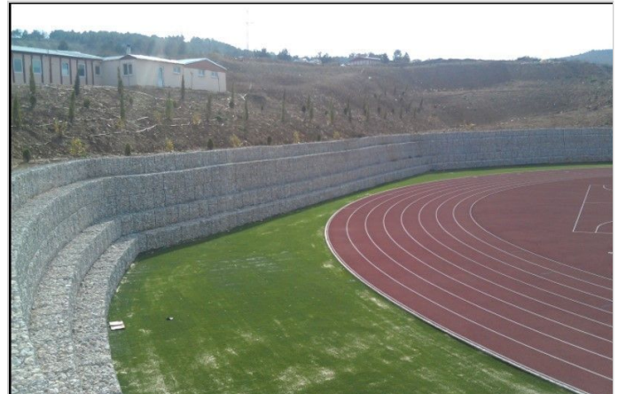
Box Gabion Retaining Wall
