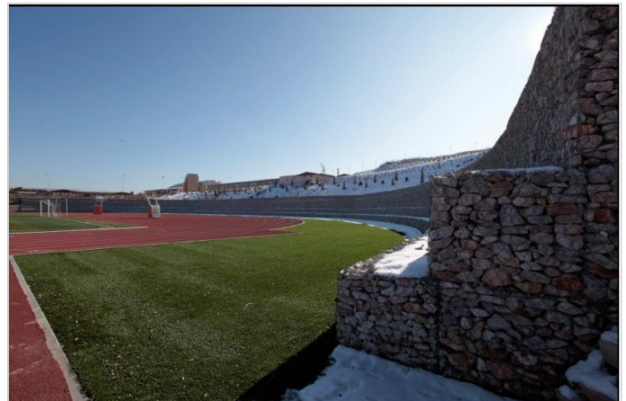
Box Gabion Retaining Wall
