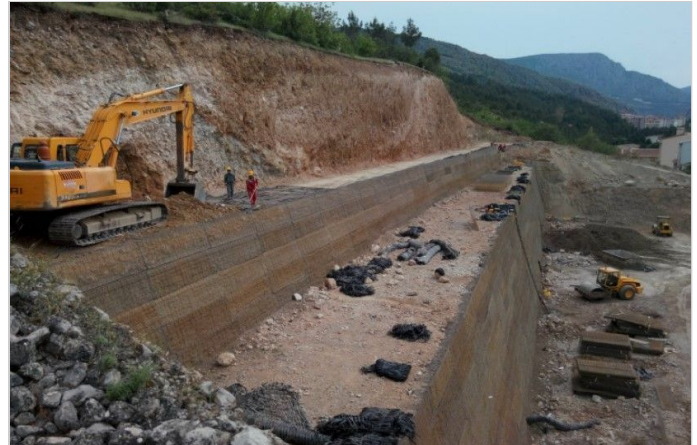
Green Terramesh Retaining Wall Construction Stage
