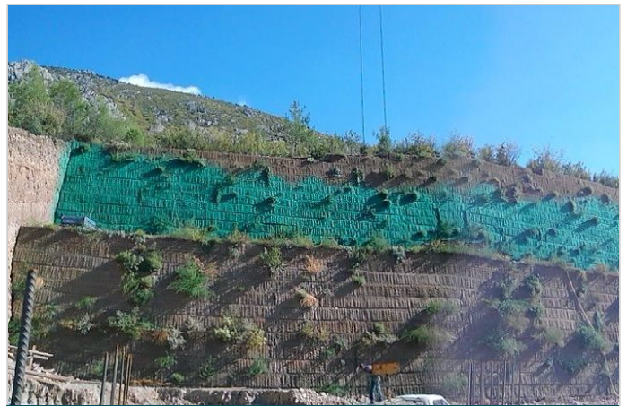
Green Terramesh Retaining Wall
