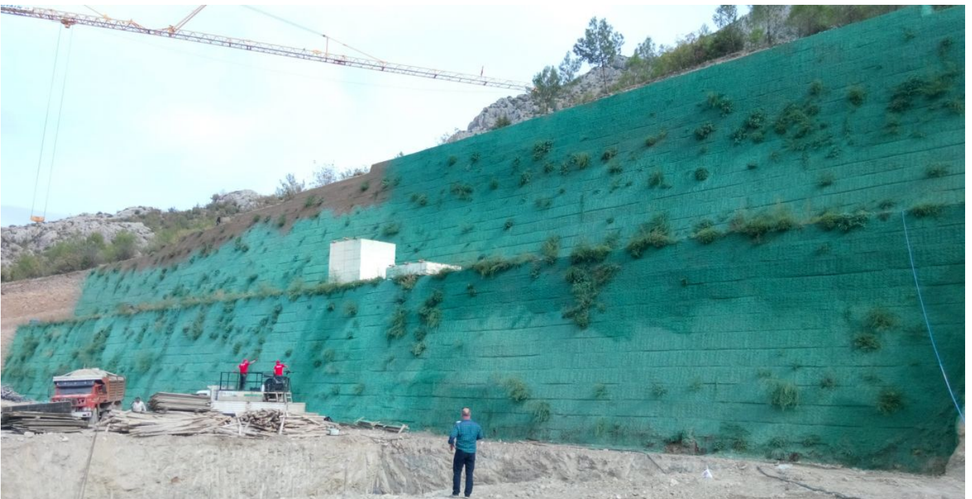
Green Terramesh after Hydroseeding
