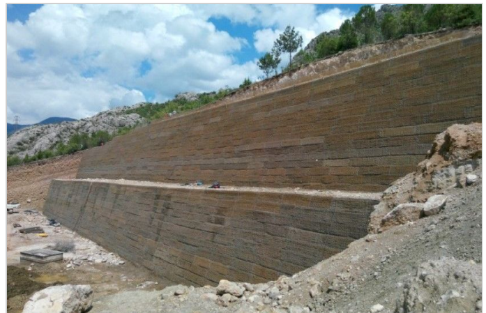
After The Green Terramesh Retaining Wall Construction
