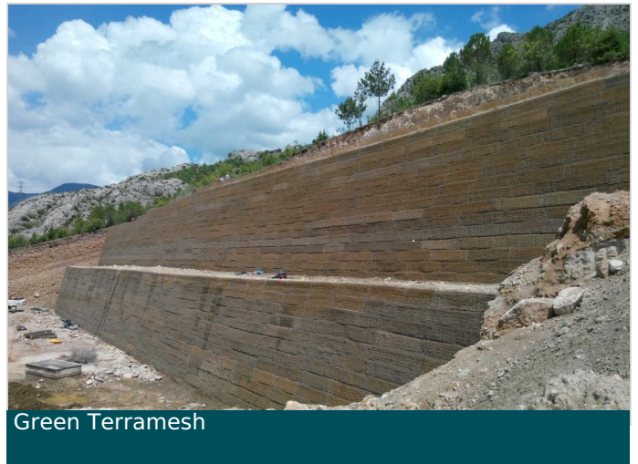
Green Terramesh Retaining Wall
