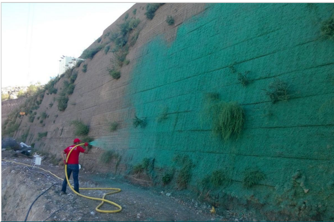
Green Terramesh Retaining Wall Spray Grass Application
