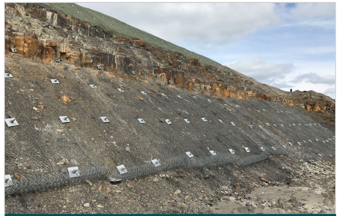
View of the slope with the Steelgrid HR 100
