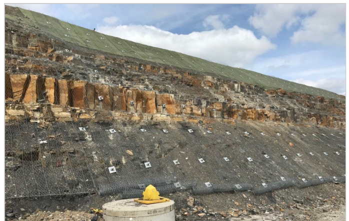
Steelgrid HR system secured to the rock face with
