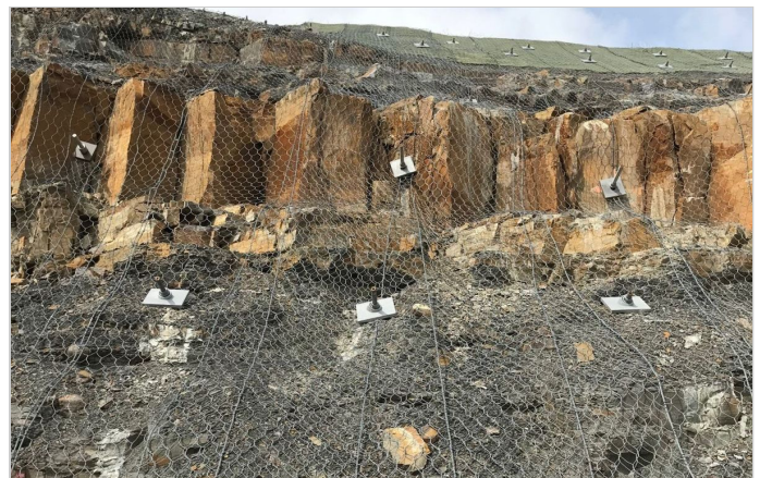
Steelgrid HR draped over the rock face
