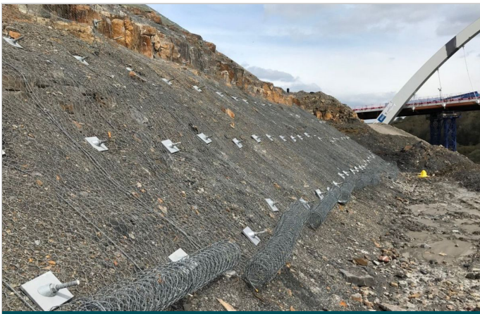
Neat mesh installation. Bottom of the rolls yet to be secured
