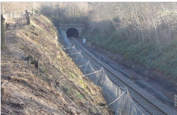
Catch fences installed on the Cumberworth Tunnel line
