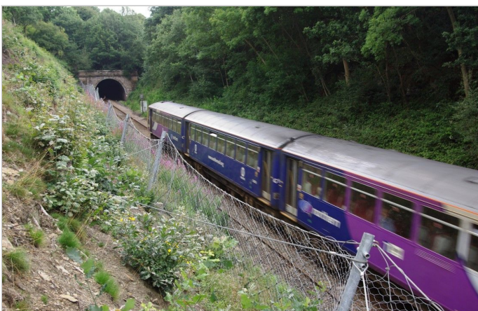
Post installation of the catch fences at Cumberworth
