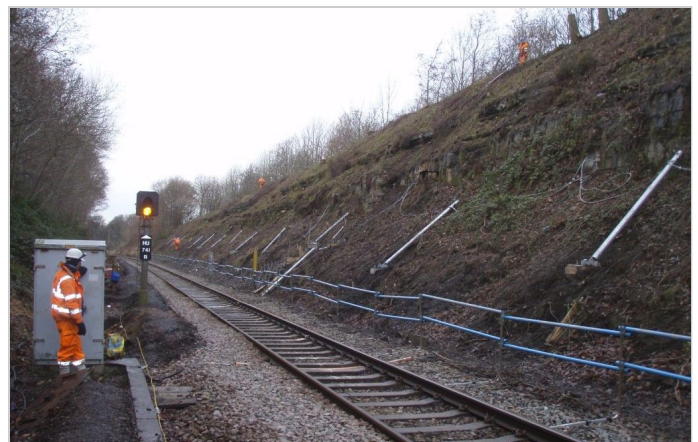
Catch fences being installed on the Cumberworth Tunnel line
