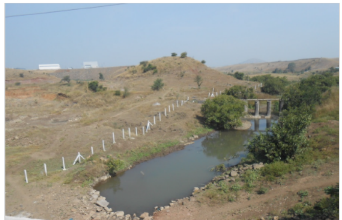
Photo 1 : Site before construction
