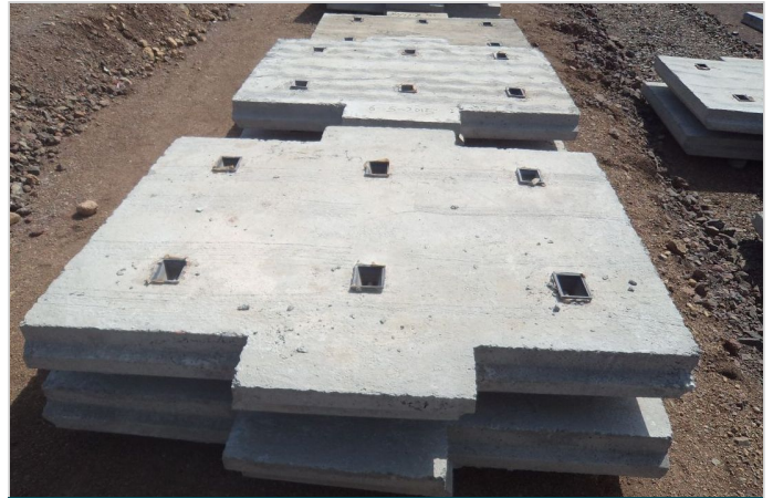
Photo 4: Concrete panel with cavity connector (MacBox)
