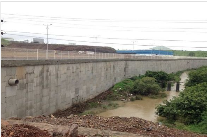
Photo 5:Complete MacRes structure
