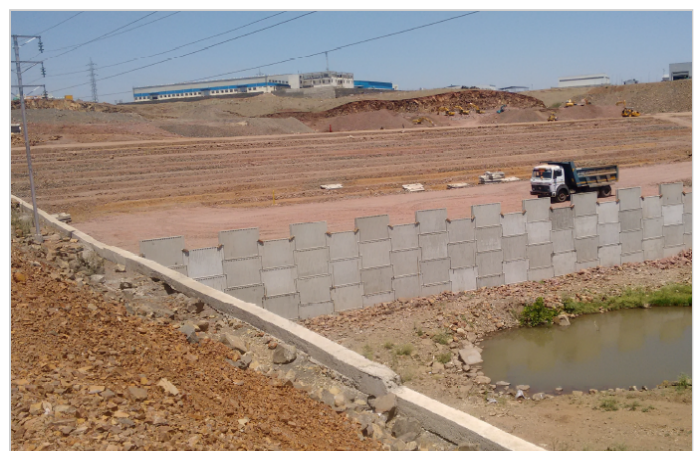
Photo 2 : RS wall under construction adjacent to Nallah
