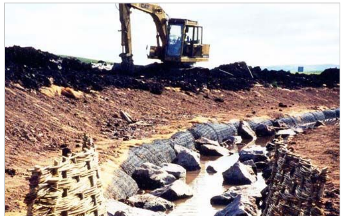
The new two stage channel during construction
