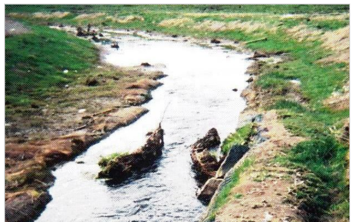
Two stage channel immediately after construction
