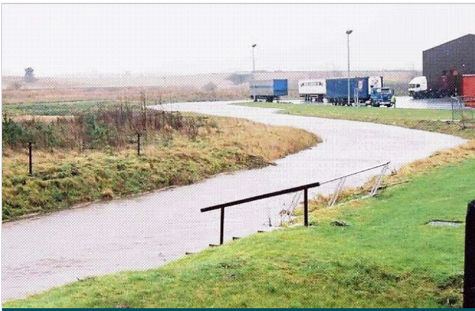
Diverted water course around new warehouse & car park
