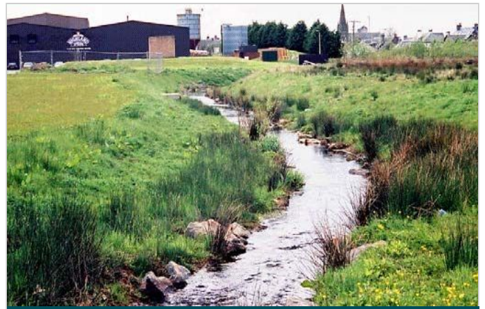
2 Years post construction showing 2 stage channel
